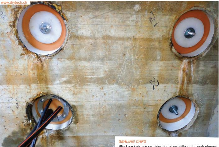
Blind gaskets are provided for pipes without through elements, also made to measure.
