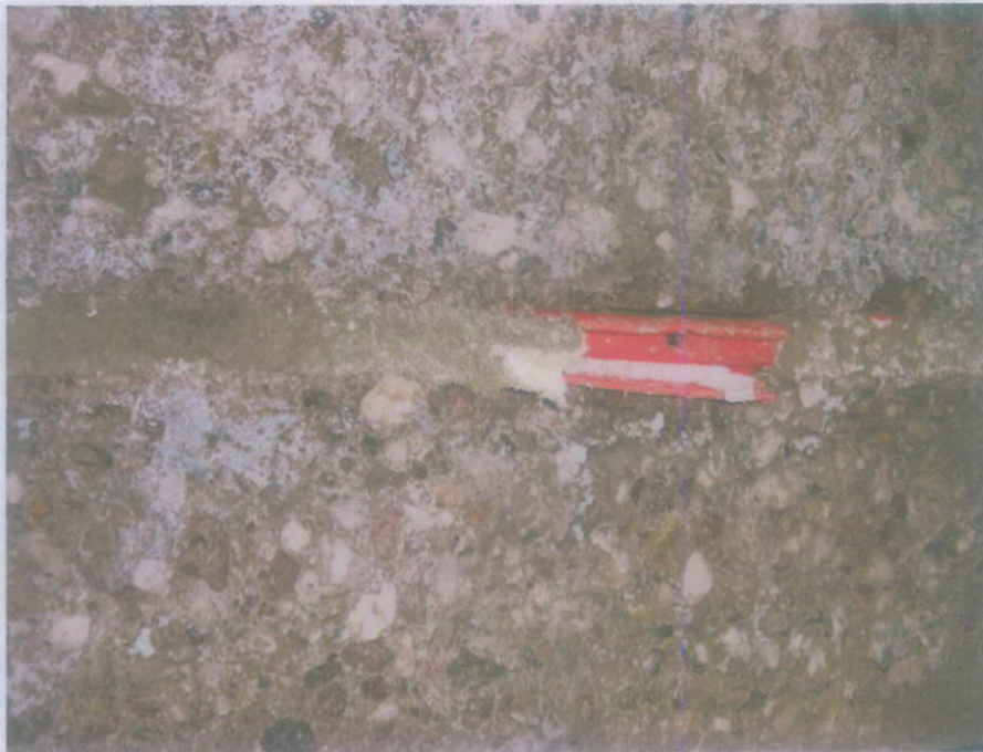
Fig. 8: Exposed injection profile after disassembling the wall frame where the distribution of the DRYflex 2 / DRYflex plus can be easily seen
